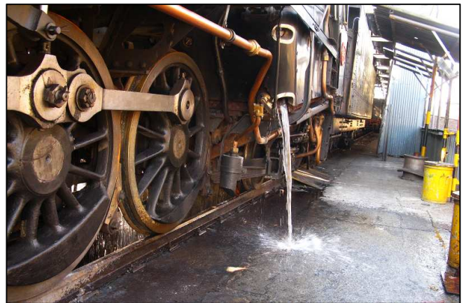
P06 - Early stage of boiler washout in progress. The fellows had yet to start raking out the foundation ring area.
