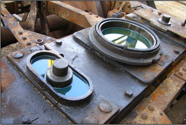
P03 - The newly repaired boss now holds oil as designed. Square-section graphite packing was installed as a seal.
